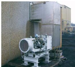
Ambient plant air is pulled into the Englo Extractor by its integrated impeller, cleaned, and then exhausted into the MCC Room.
